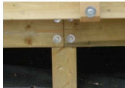
Deck and boardwalk support BSEN335:1 Use class: 4 (for posts), 3.2 (for for beams and joists out of direct ground contact)
