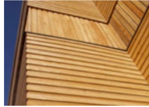
External timber cladding
